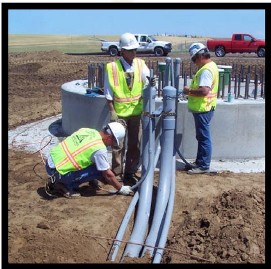
Conduit installation at wind turbine foundation. Photo credit: John Demoss
