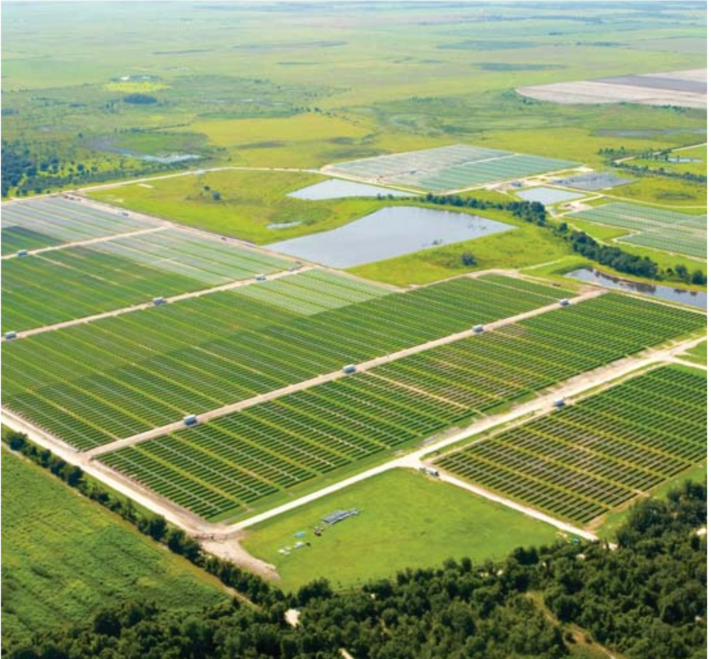
Photo courtesy Florida Power and Light
